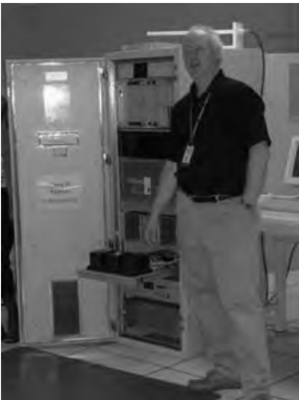
Automated Surface Observing System (ASOS)
